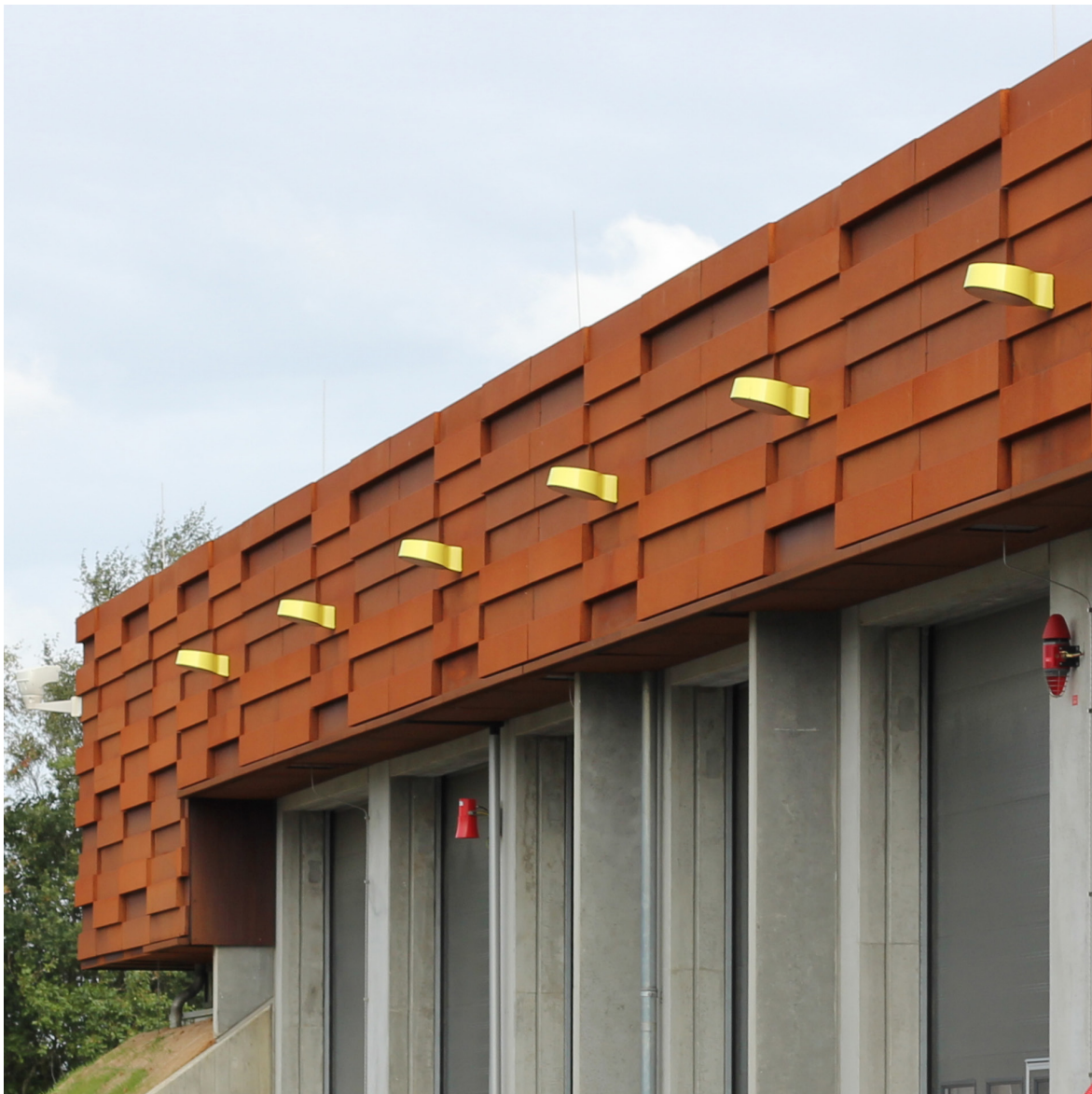
Egtved Gas Compressor Station, architects: C.F. Møller
